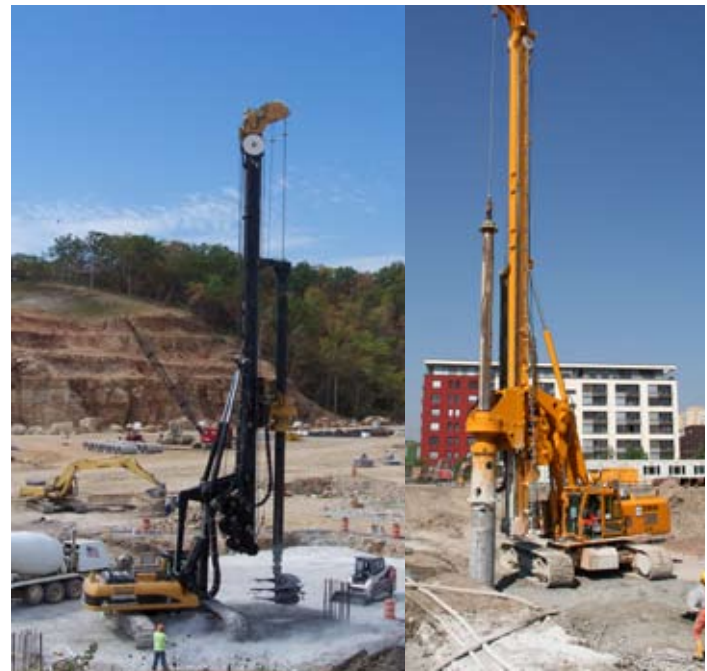
RH26 Kelly drilling without casing
