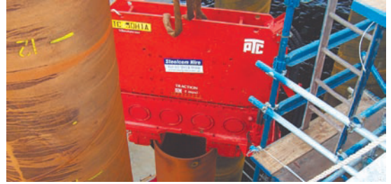
Crane suspended vibrators
