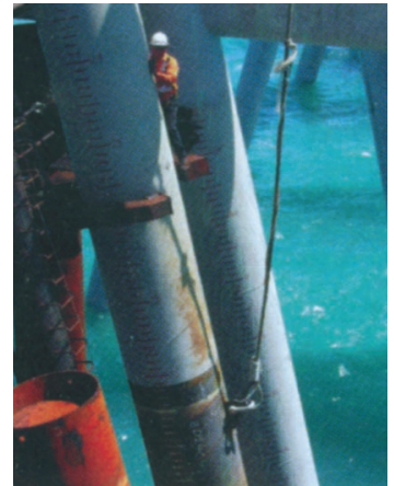
Close up view of 40m long steel tube piles
