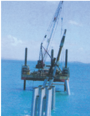
9t BSP 357-9 hammer driving steel tube pile into the seabed
