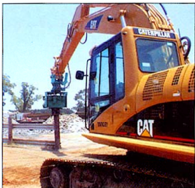
35ft timber piles being driven in US
