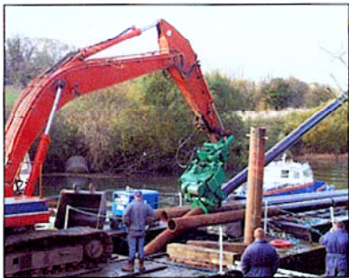
Manipulating steel piles on a barge
