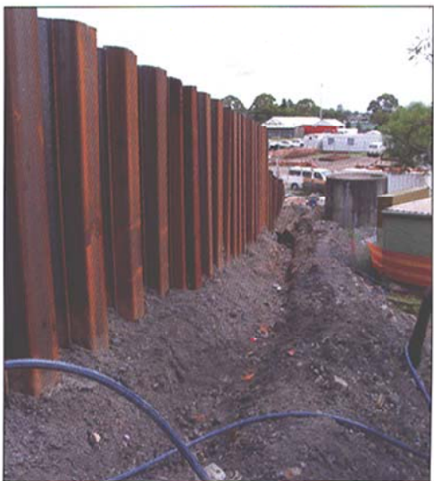
Wall of sheet that will be shotcreted and remain permanently exposed.
