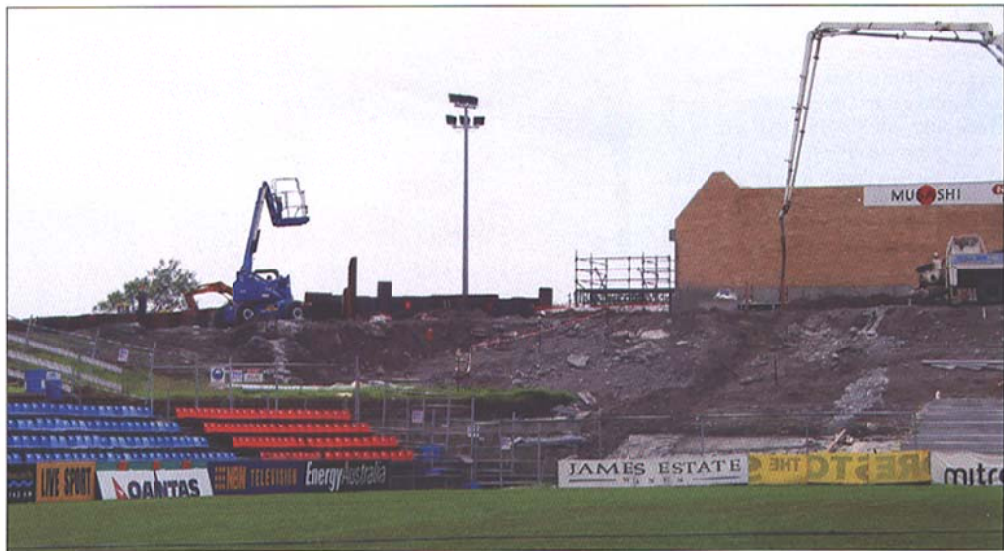
A new grandstand is being constructed at EnergyAustralia Stadium in Newcastle.
