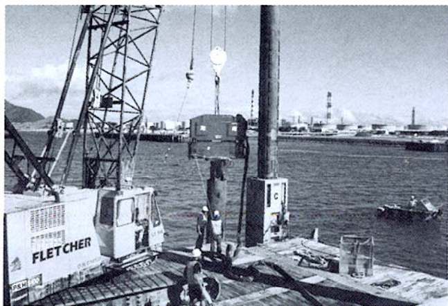
Steelcom's 50HL hammer in operation at Marsden Point.
