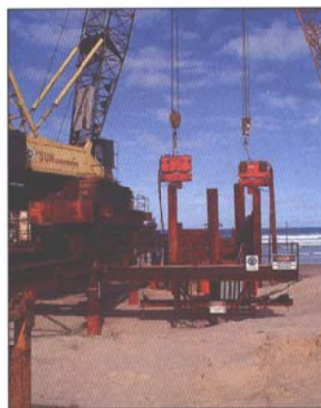
PTC 25H2 and 30H1 vibro-hammers were deployed to drive sheet pile.
